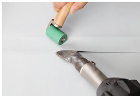
The plastified lap areas will be fused by applying moderate pressure with a silicone pressure roller, following parallel to the opening of the nozzle. Due to the backwards movement, the nozzle always blows against already seal welded areas of the seam.
