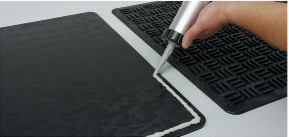
It is recommended to install the tiles with a joint spacing of more than 50 mm. alwitra EVATAACK may be visible at some parts along the edges. One cartridge will bond approx. 3 maintenance walkway tiles.
