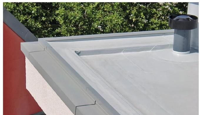
Note: With the flashing against the roof sealing being set back by 120 mm, rainwater in this area will drain off over the front surface of the profile!
