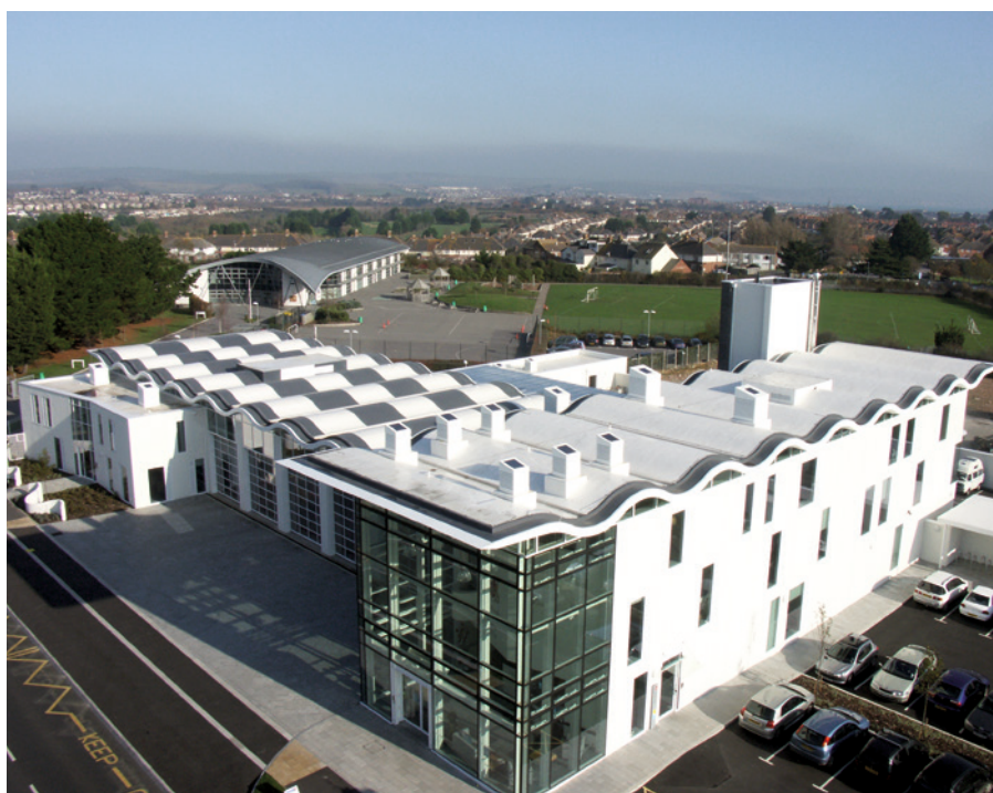
Fire Station, Weymouth, England
