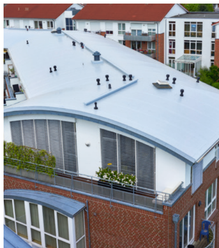
Residential building complex, Meppen, Germany
